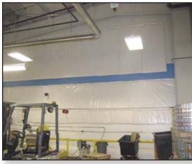
Fiberglass absorbers reduce the reflection of sound waves by adding soft, porous, open-celled materials to an environment. The Sanitary Acoustical Baffle is durable, low cost and virtually rip-proof. The sound absorption core is completely encapsulated in reinforced mylar film. The white facing reflects light, which adds to the illumination in a room. Wall panels are constructed with all edges bound and grommets across the top.
