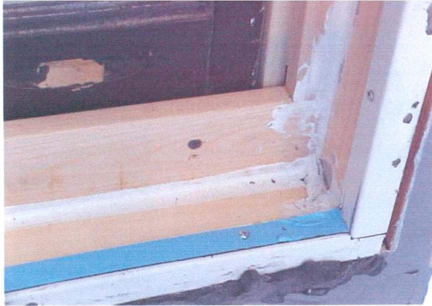
Sheet Metal Angle Mounted to Test Sample for Frame Mount Application
