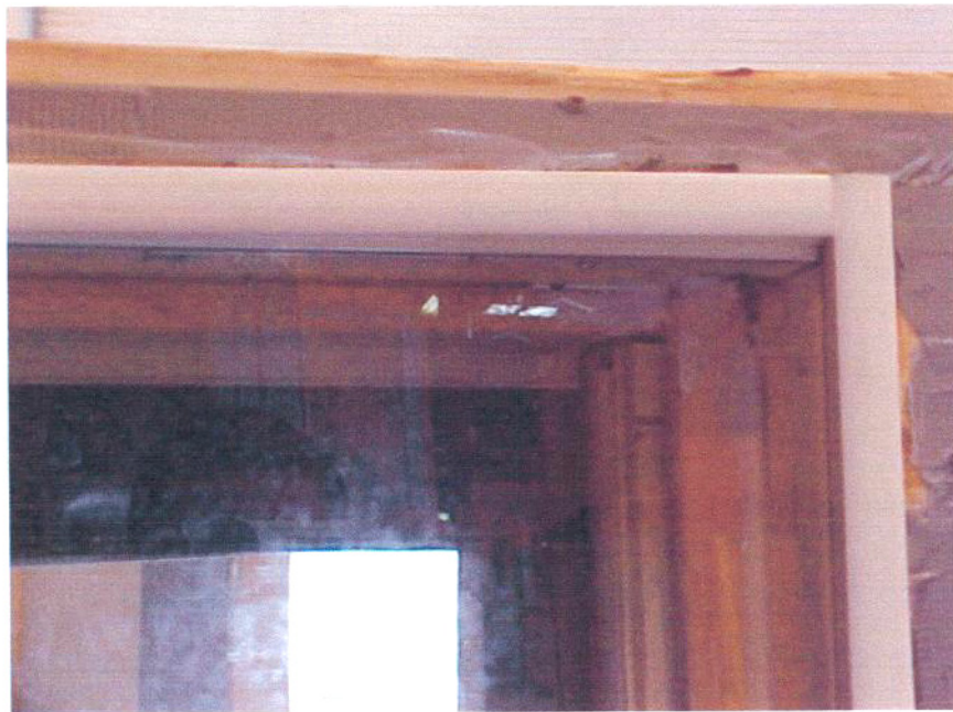
Frame Mount Storm Window Installed onto Sheet Metal Angle
