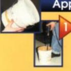
To prepare the glue mixture, read the manufacturer's instructions because, once it is mixed, there is very little time to apply it. Wear gloves to avoid all contact.
