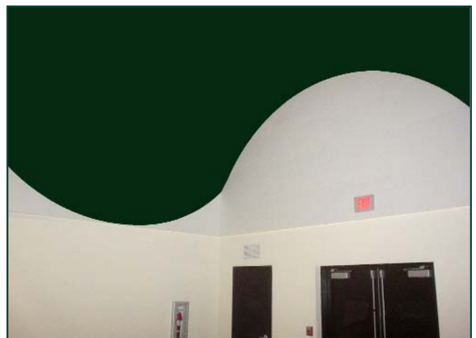
There is a smooth transition of the wave from two perpendicular walls.
