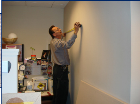
These panels were installed with our two-part E.C. Clip. One part of the clip is epoxied and screwed into the back of the panel, the other part of the clip is screwed to the wall.
