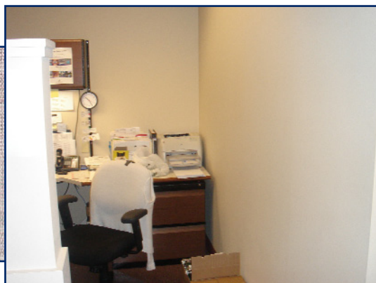
The work stations in this office were constructed almost exclusively out of sheetrock which did not offer anywhere for the sound from a normal conversation to be absorbed.
