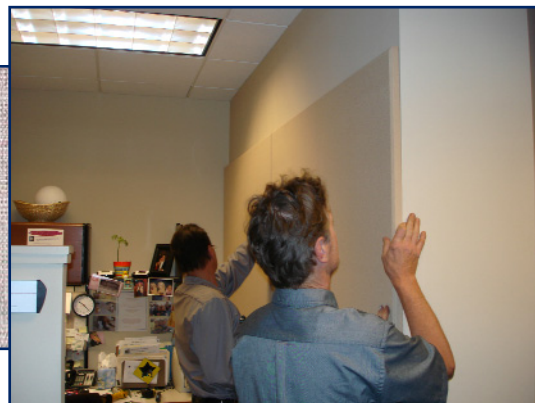
I had the outer edges of each panel chemically hardened so that the fiberglass core would not break down and dent in case someone hit the panel with their shoulder when they turned the corner to her work station.
