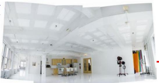
coustical Surface's Echo Eliminator B.A.P. (Bonded Acoustical Pad) recycled cotton acoustical panels solved the reverberation problem while maintaining the existing aesthetic of a photography studio in the heart of New York City. The studio is in a solid concrete building in which the ambient noise level of the space was decreased from 55 dBa to 44 dBa.
