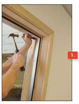
2. A Install sealant backer rod into space between doorjamb and rough opening a minimum of 1" deep. B Squeeze in acoustical sealant.
