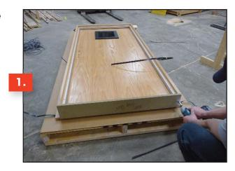
Verify door swing and stand door against wall on appropriate side. Verify rough opening width and height.
