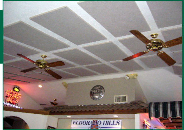
1" Beige Echo Eliminator™ throughout the ceiling was used in a checkered pattern.
