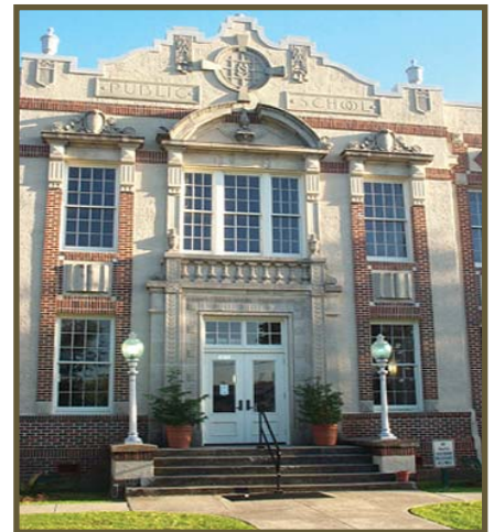
Historic Schoolhouse 2nd Floor Sound Studios.
