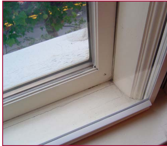
Climate Seal™ Acoustic Series window insert applied over existing storefront glass for maximum sound protection from street traffic. Ipswich, MA.
