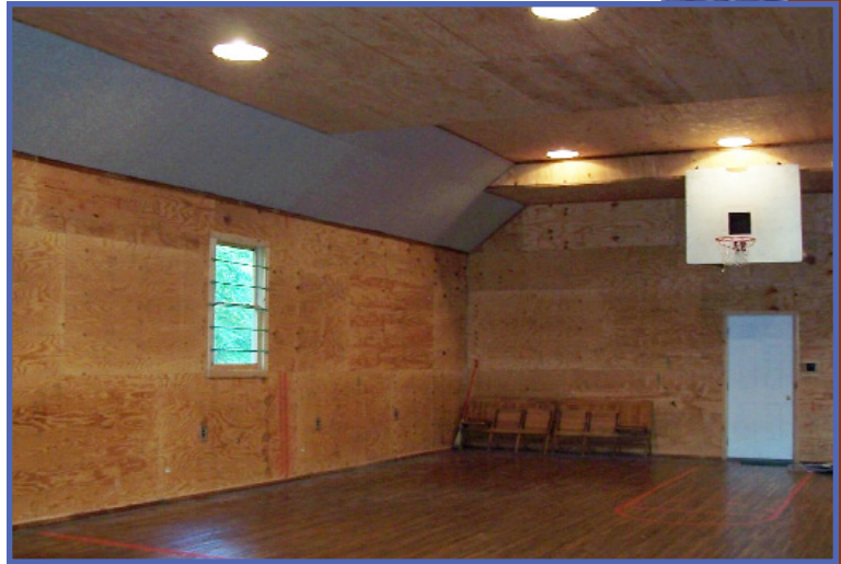
The acoustical panels were put on the angled part of the ceiling because the location was an even balance of ease of installation.
