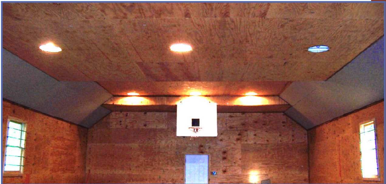
The calculation that I used for the square footage at the Central Advent Church was as follows: The room that they were considering was approximately 40' x 26' x 19' average ceiling height, or approximately 19,760 cubic feet of volume. If I take three-percent of that, I am left with 592.8, which I rounded up and converted into a square footage of panels needed.
