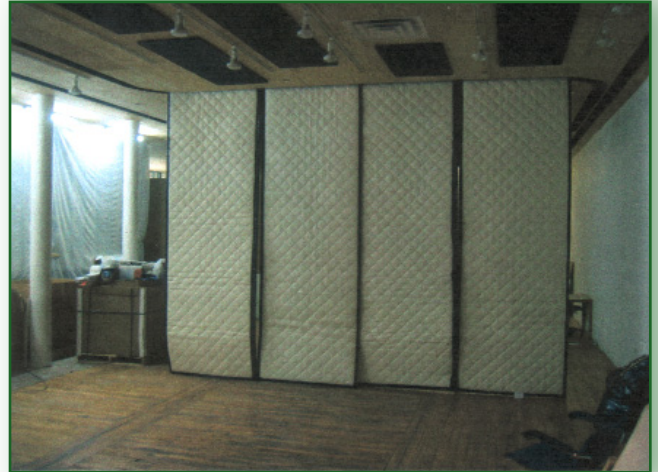
Black Nexxus Studio under construction.
