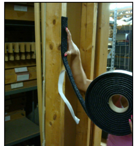
Install without mess. Screw drywall to studs through Acousti-Gasket Tape.
