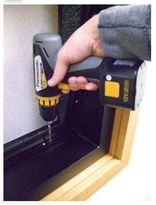
**3.** Predrill holes in frame through glass channel as shown at shim locations.
