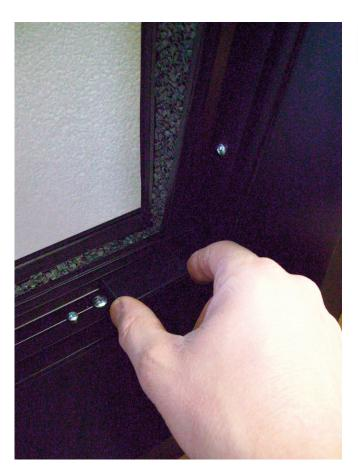
**1.** Place rubber setting pads on bottom surface of the glass channel about 4" in from the corners. (Some glue or two-sided tape will help hold them in place during glass installation).
