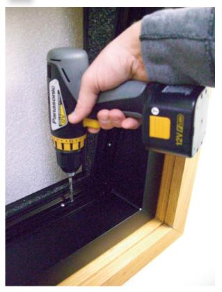
**3.** Predrill holes in frame through glass channel as shown at shim locations.
