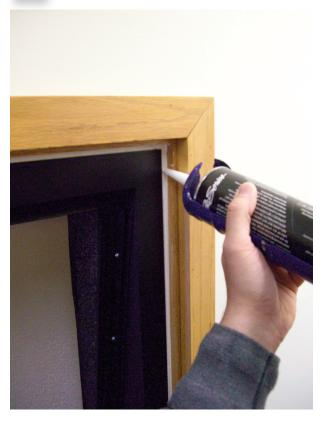
**6.** Fill the gap with acoustical sealant between window frame and opening on all four sides completely to eliminate any sound leaks.
