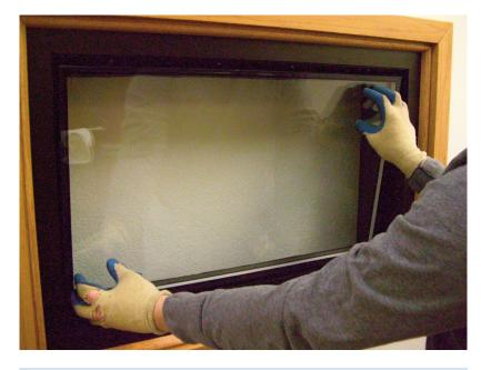
**2.** Wearing gloves and/or using suction cups, lift the glass into place and rest the bottom edge on the two setting pads and up against the rubber seal on the inside of the window jamb. Gently tilt the top of the glass into place making sure it is centered in the opening.
