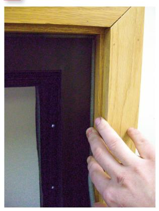
**5.** Apply sealant backer material between the outside of frame and wall opening. Recess 1" into gap to allow space for acoustical sealant.
