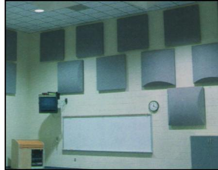
**MATERIAL:** Gel coated or fabric faced molded fire retardant resin reinforced glass fiber.
